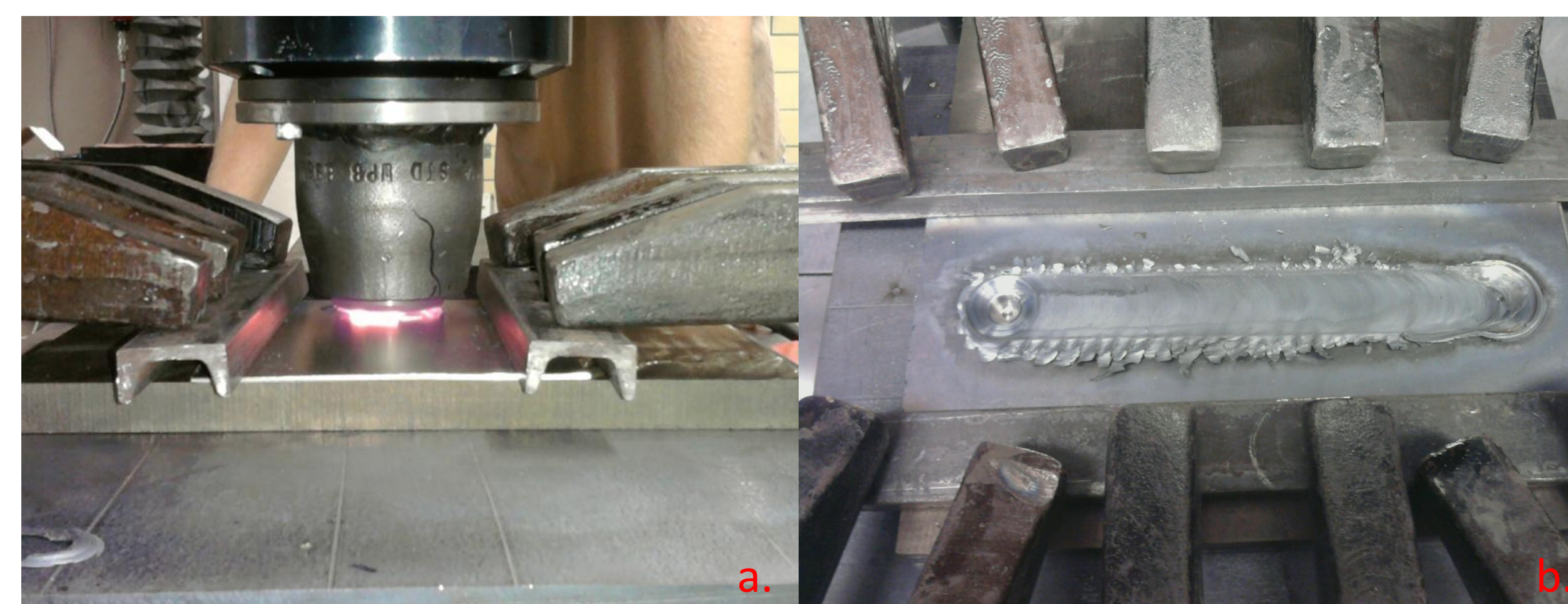
Fig. 3: (a.) Welding of cast iron with steel cover plate (b.) finished cast iron weld.
